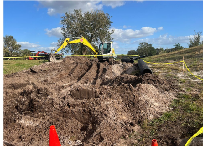
18" ADS Replacement (Lancaster 1)
