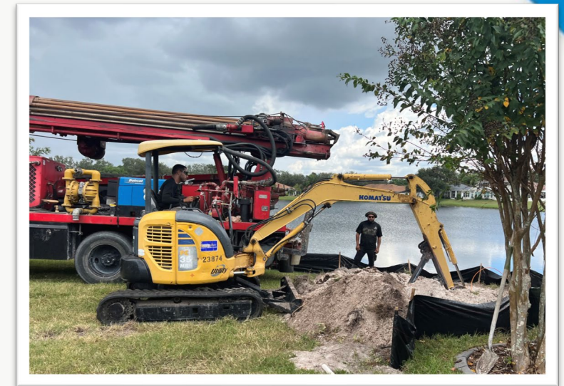
Recharge Well Drilling at Oxford
