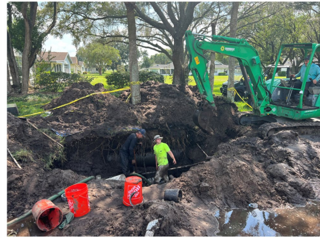
6" Mainline Repair on Hammersmith
