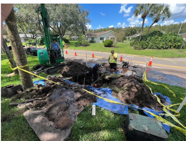
6" Mainline Repair on Hammersmith
