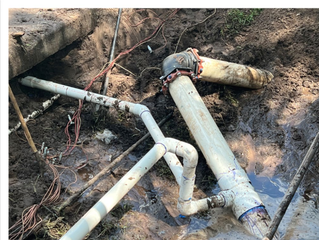
6" Mainline Repair on Hammersmith
