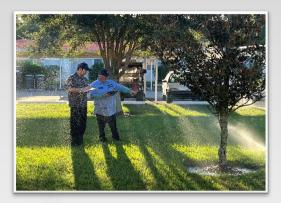
Perform visual inspections of each irrigation zone running in the same programming environment that each particular zone is normally scheduled to run on. Programming for each zone will be provided by the Master Association's Water Manager.
