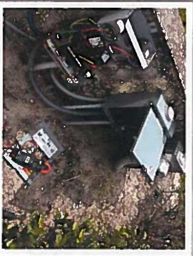
Pump Control Box Replacement Inverness
