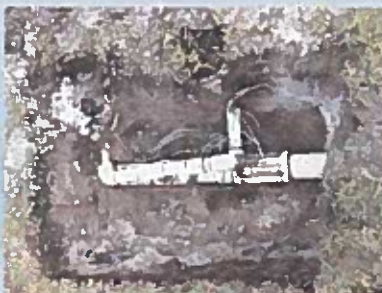
Gloucester 6" Mainline Repair
