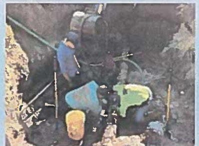
Hammersmith 8" Mainline Repair
