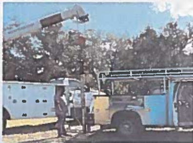
Upper Loop 40Hp Pump Replacement
