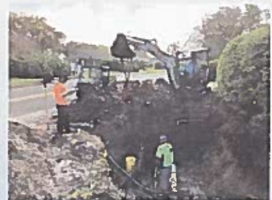
Hammersmith 8" Mainline Repair
