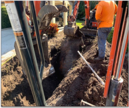
30" Storm Pipe Replacement Finsbury Cr.
